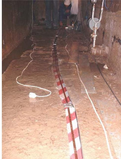
Figure 8: SMARTape installation in the inspection gallery.
