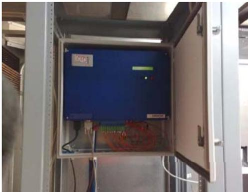
SOFO Fiber Optic Sensor Datalogger
