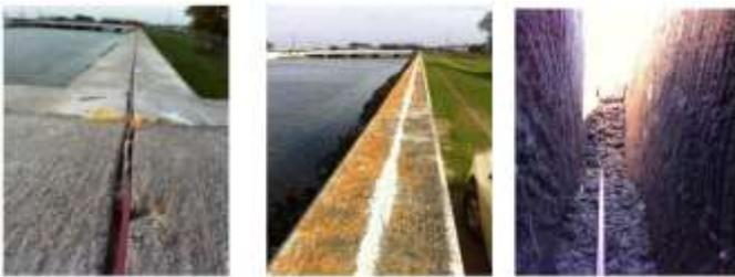
Figure 7. Installation of sensor in a groove, on top of the levee wall section and in a trench
