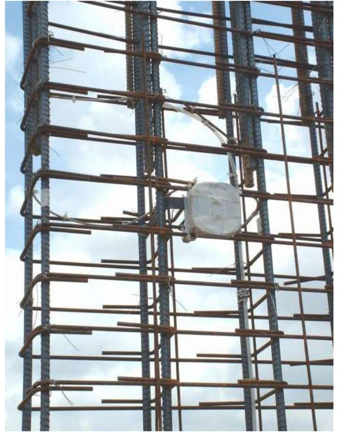
Figure 3. Long-gauge fiber optic sensor and junction box in a column before concrete pouring
