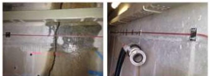
Figure 10. Strain sensing cable installation on penstock access tunnel
