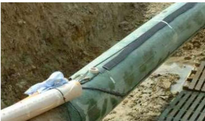
Figure 12. Strain sensing cable installation
