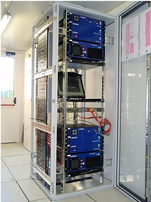
Figure 1: Fully redundant leak detection system
