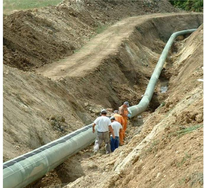
Figure 8: SMARTape on the gas pipeline.
