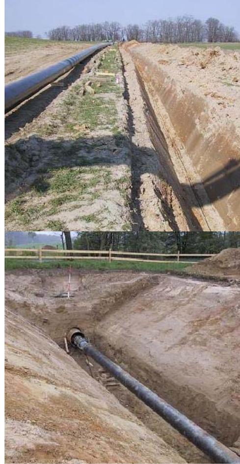
**Figure 6. Construction phase of a buried brine pipeline in the north-east area of Berlin. The fiber optics cable is placed in the sand at the 6 o'clock position about 10 cm underneath the pipeline.**
